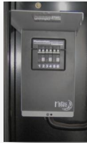
Figure 15 Combiner/ Breaker box, accessing breakers
