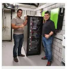
20KVA 3PHASE 50KWH Lifepo4 Battery HYBRID Solar Energy Storage System
