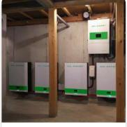
8KVA hybrid inverter 40kwh powerwall in Japan
