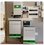
5KVA hybrid inverter 20kwh powerwall in Africa
