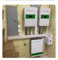
16KVA hybrid inverter 10kwh powerwall in Germany
