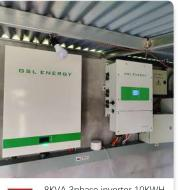
8KVA 3phase inverter 10KWH solar system in Switzerland
