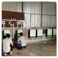
10KVA single phase inverter 40kwh powerwall in Myanmar
