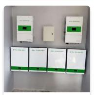
16KVA hybrid inverter 40kwh powerwall in Jamaica
