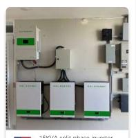
15KVA split phase inverter 30kwh powerwall in USA
