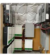
48KVA split phase inverter 70kwh powerwall in USA
