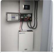
8KVA split phase inverter 10kwh powerwall in USA
