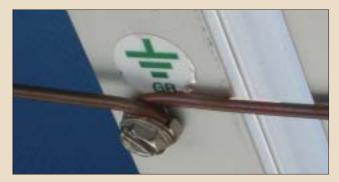
Photo 5. Improperly installed grounding hardware
