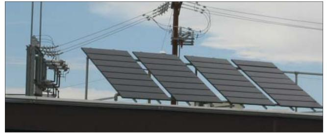
Photo 2. Utility-interactive PV system under power lines
