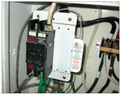
Photo 6. External ground-fault protection device
