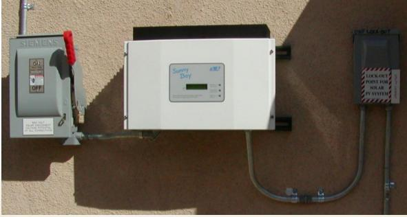
BOS: The balance of the equipment necessary to integrate the PV array with the site load (building). This includes the array circuit wiring, fusing, disconnects, and power processing equipment (inverter).
