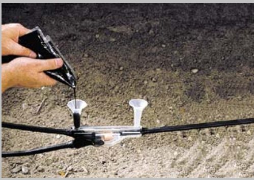
Exhibit 300.9 An underground splicing method. (Courtesy of 3M Co., Electrical Markets Division)
