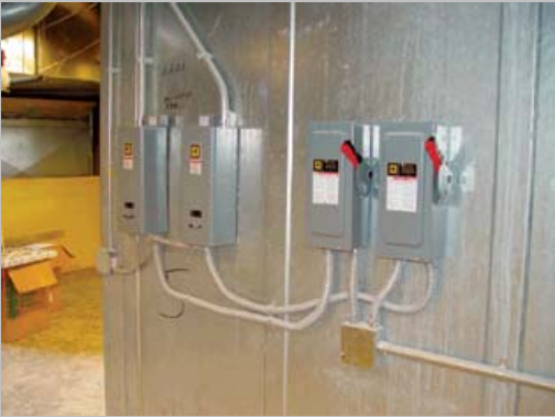
Exhibit 430.18 The disconnecting means for each controller, which must be within sight of the controller location. (Courtesy of International Association of Electrical Inspectors)
