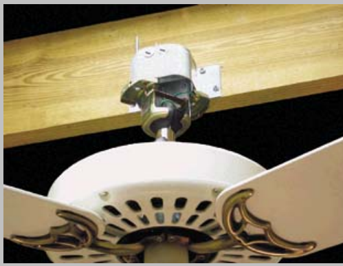
Exhibit 422.2 Supporting a ceiling-suspended (paddle) fan (35 lb or less) with a box identified for such use. (Courtesy of Hubbell RACO)
