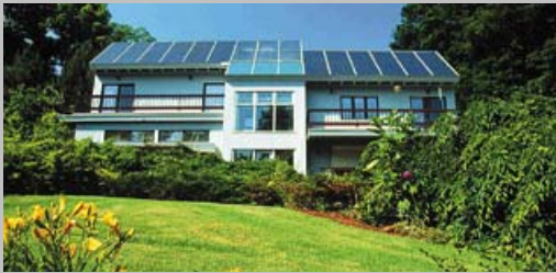
Exhibit 690.1 The south roof of a solar house. The integrated array of glass modules generates electricity directly from the sun using PV modules. (Courtesy of Solar Design Associates, Inc.)
