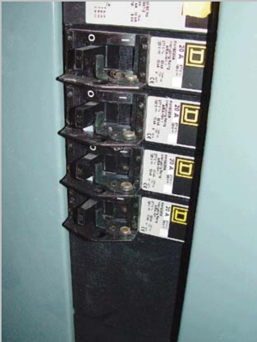
Exhibit 440.1 Four circuit breakers equipped with locking hardware that is not readily removable or transferable. (Courtesy of International Association of Electrical Inspectors)
