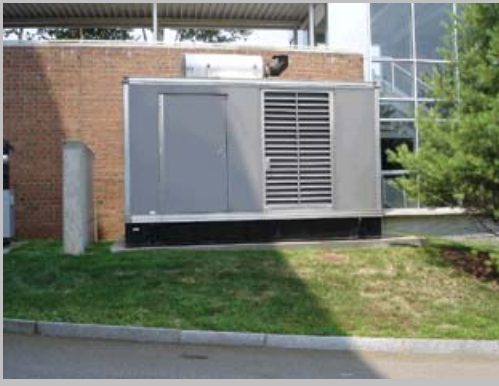
Exhibit 700.2 Alternate source of power in a heated and secure building that is located in an area not subject to flooding.
