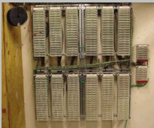
Exhibit 800.3 An example of punch blocks used on a private automatic branch exchange.
