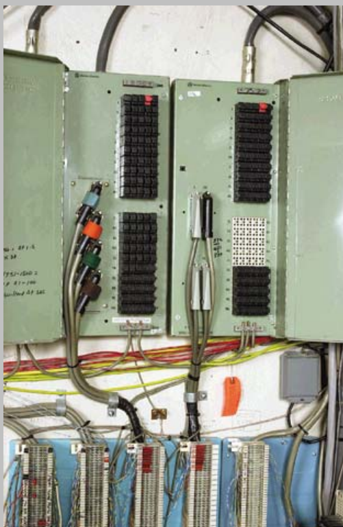
Exhibit 800.4 A primary protector unit typically installed in commercial buildings. This unit is the interface to the outside plant cable.
