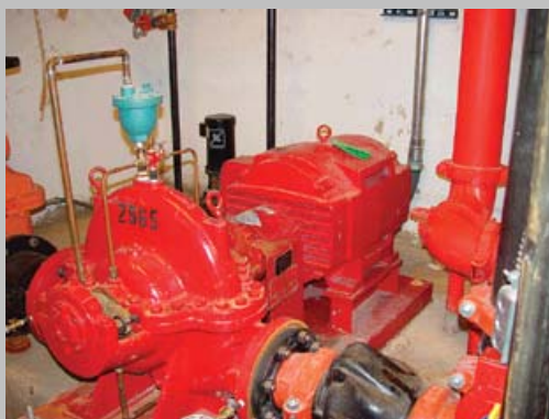
Exhibit 695.1 An electric motor specifically listed for fire pump service. (Courtesy of International Association of Electrical Inspectors)
