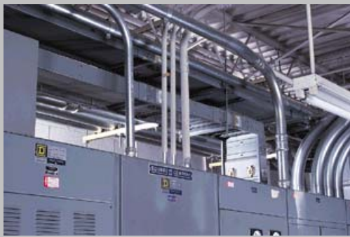
Exhibit 368.1 A 10-ft section of feeder busway.
