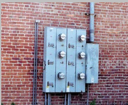
Exhibit 230.26 An enclosure for grouping service equipment consisting of six circuit breakers or six fused switches.
