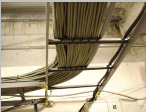
Exhibit 800.7 Overhead ladder-type cable tray containing communications cables.
