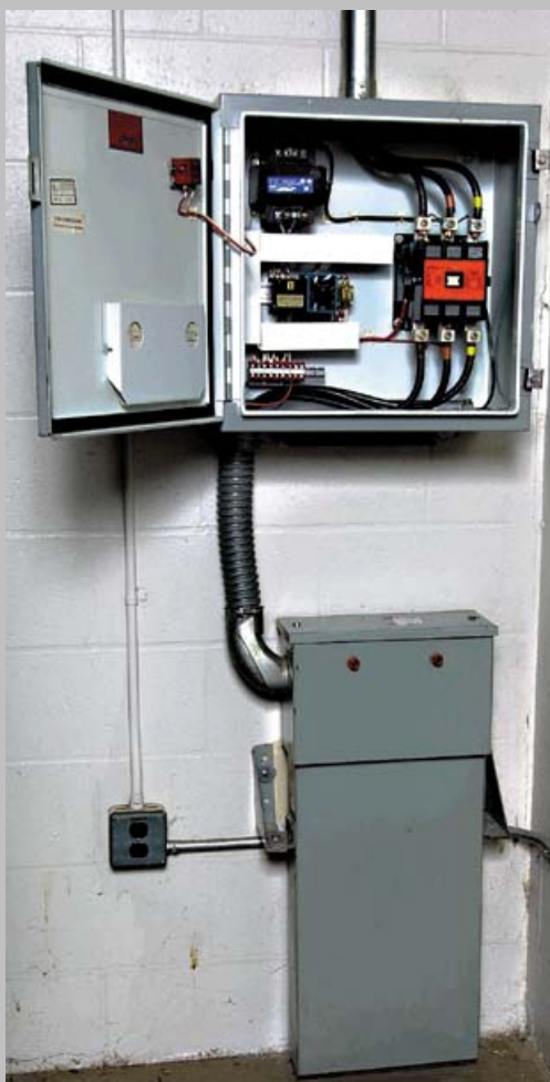
Exhibit 460.2 Power factor correction capacitors with discharge resistors.
