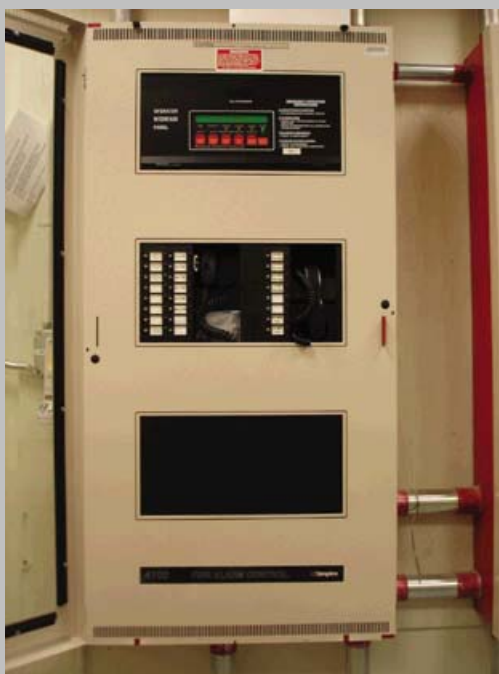
Exhibit 760.1 Typical fire alarm control unit.
