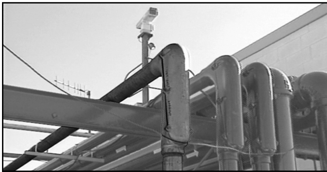
TYPICAL CLASS I, DIV. 2 RIGID CONDUIT INSTALLATION.
