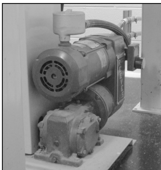
TYPICAL CLASS I, DIV. 1 WIRING.
