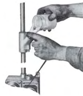
MIX KWIKO SEALING CEMENT THOROUGHLY IN A CLEAN CONTAINER. POUR DIRECTLY INTO THE SEALING FITTING. DEPTH OF SEALING COMPOUND SHOULD EQUAL TRADE SIZE OF CONDUIT, HAVING A MINIMUM OF 16 MM (5/8 IN.) THICKNESS.
