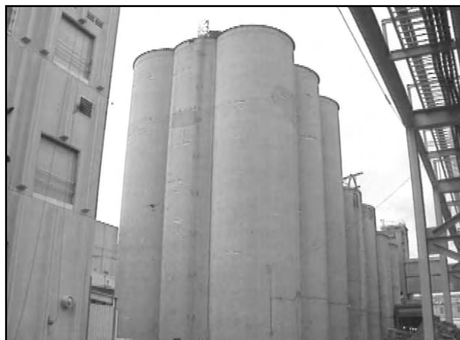
GRAIN ELEVATOR—CLASS II, DIVISIONS 1 AND 2.
