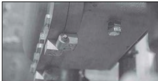
ECDB DRAIN INSTALLED IN BOTTOM OF EXPLOSIONPROOF ENCLOSURE.
