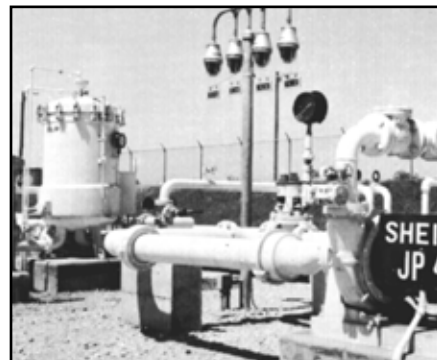
INSTALLATION OF LUMINAIRES IN JET FUEL AREA.
