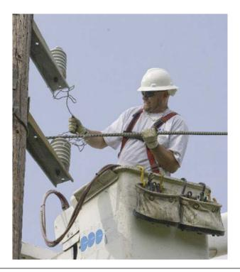
**Figure 8.7** Line workers are required to adhere to approach minimums and inadvertent movement allowances.
