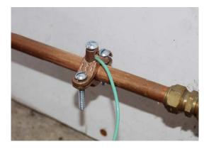
Figure 5.2 Copper water pipe can serve as an effective ground-fault current path.
