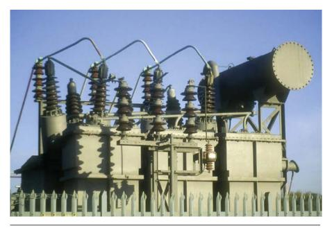
**Figure 8.3** A voltage transformer is used to convert high voltage supply current to a lower voltage.
