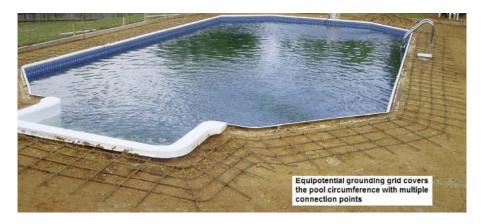
**Figure 6.8** An equipotential grounding grid protects anyone getting out of the pool from shock hazards because they would have the same electrical charge as the pad.
