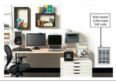
Figure 9.9 Office heater loads must be based on the total current draw of all the heaters.
