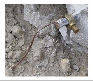
Figure 5.12 A bonding jumper attached to rebar which is encased in concrete.
