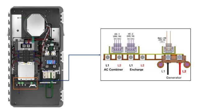
Figure 10: Enlarged view of generator lugs and auxiliary contact.
