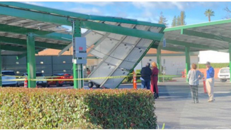
This structure collapsed after suffering wind damage.
