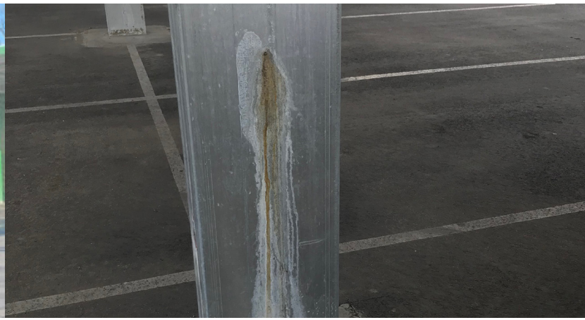
This structure is showing significant signs of corrosion only 1 year after being installed.
